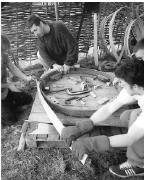
Bending the wheel on the former.
