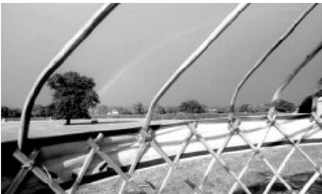
Roof ribs, trellis and band.
