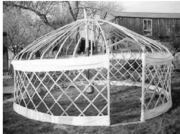
The completed yurt frame erected.
