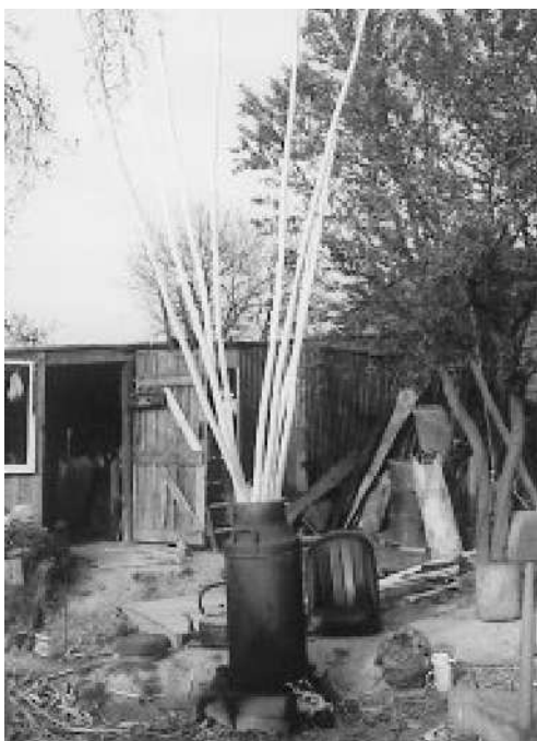
Boiling the ends of roof ribs.
